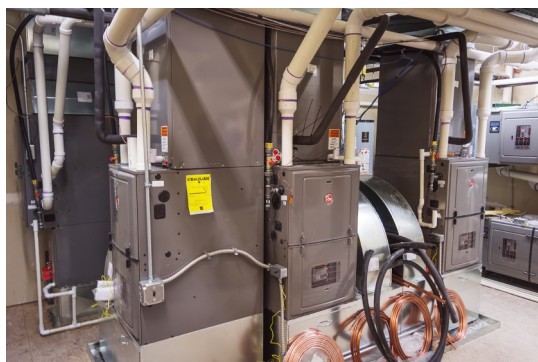
Three newly installed Rheem heating and cooling units (foreground), and a fourth at background left, located above the kitchen and off the sound room, are shown on Friday evening, April 15. The three foreground units, when fully operational, will regulate temperature in Fellowship Hall. The looped-copper tubing on the floor will provide refrigerants.
